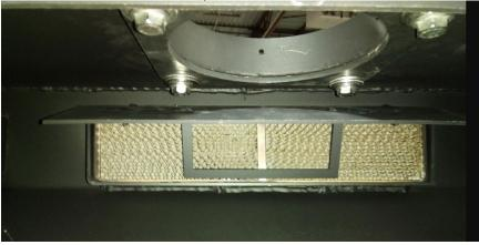
**Step 3:** The blocker plate that was removed from the rear of the stove can then be inserted over the opening at the top of the stove, the spacer plate placed below, and the entire assembly secured to the top of the stove with bolts ash shown below. Before tightening bolts, be sure that no gaps exist between the blocker plate and the top of the stove whereby smoke may escape. If necessary, gasket cement can be placed between the plate and the top of the stove.
