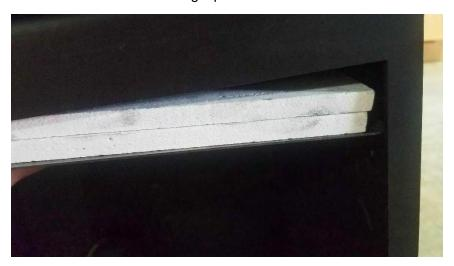
**Step 7**: While facing the pedestal, first place the metal shield and insulation directly on top of the fixed clips on the left-hand side. Next, the metal shield and insulation should be elevated above the clip holders on the right-hand side. Then, using your other hand, slide the two clips into place as shown in the pictures below. The metal shield can then be set down on top of the clips
